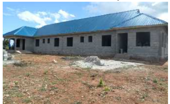
The Under Construction Guest House Visited by Annual Conference Delegates.
